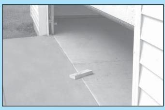
FIG. 6-6 2 x 4 under center of door opening.
